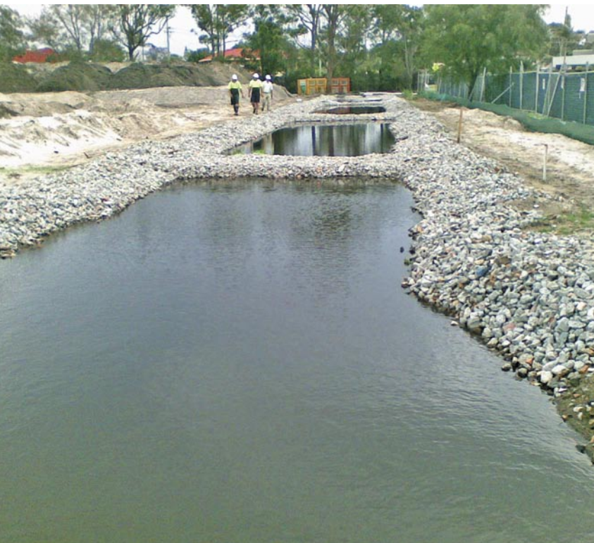
Above: Baffled retention pond at confined site.
