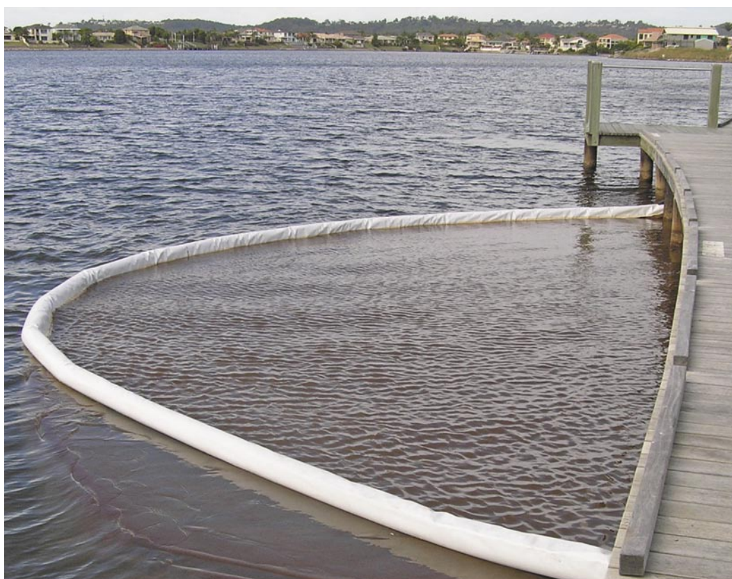
Above: Floating silt curtain providing secondary protection of receiving waters.
